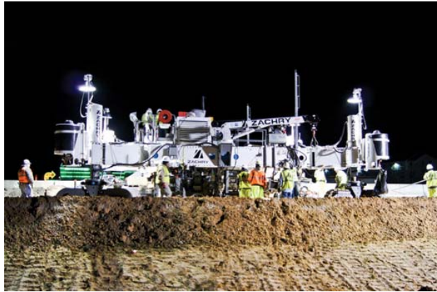
Contractor Zachry Construction has been using its G&Z paver on a contract in South Carolina
