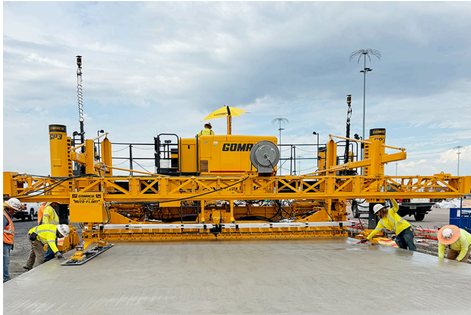
A four-track GOMACO GP3 with Topcon 3D guidance is paving on the Memphis International Airport in Tennessee.
