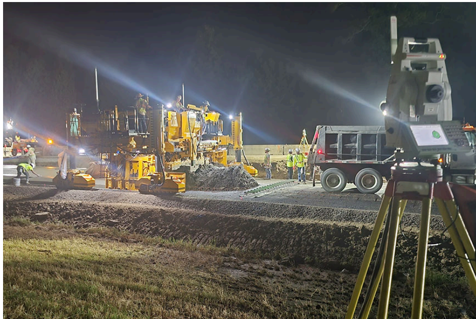
A four-track GOMACO GP3 with Leica 3D guidance is mainline paving at the I-12 and I-10 interchange in Baton Rouge, Louisiana. The mold has side-bar inserters and a spreader plow.
