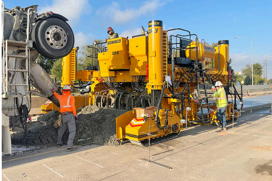
A four-track GOMACO GP3 is slipforming a concrete scab-on lane on Tinker Diagonal Street in Del City, Oklahoma.
