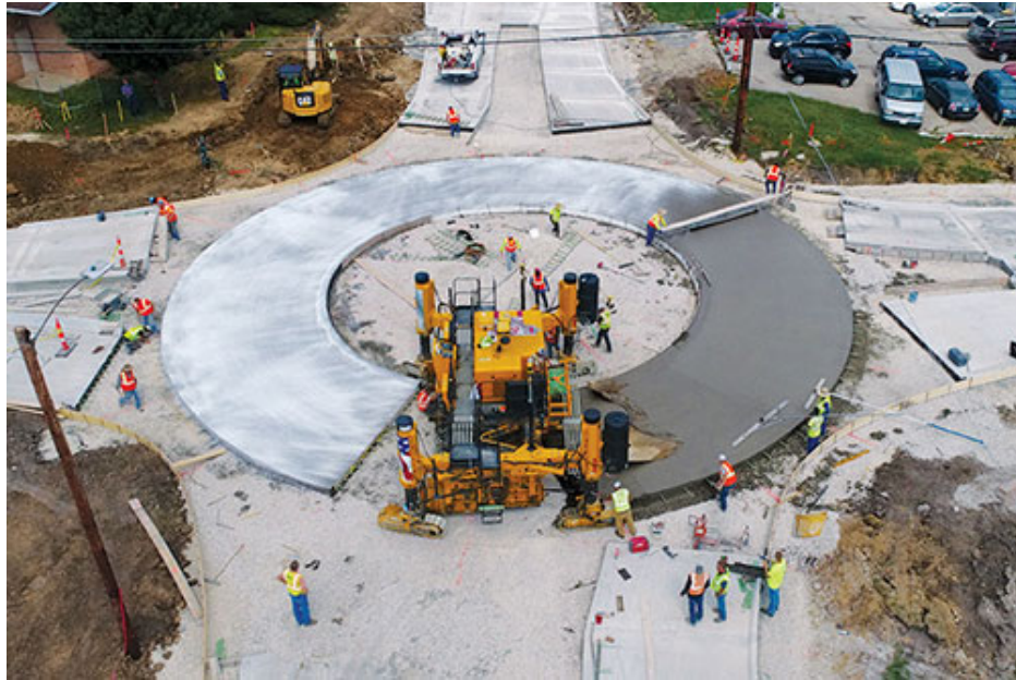
An 18 foot (5.49 m) wide roundabout with a 22 foot (6.71 m) inside radius is being slipformed by the GOMACO GP3 four-track slipform paver using 3D machine guidance.
