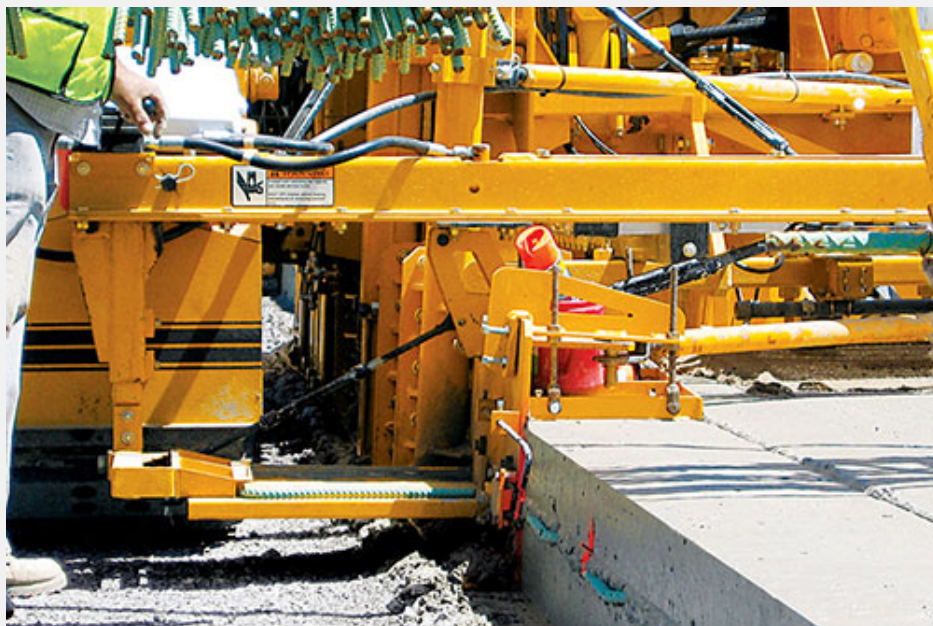
Trailing form with air-powered bar insertion.
