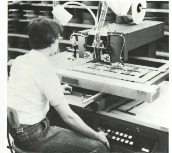
Fig. 9-3. Computer-controlled automatic insertion machine. (Courtesy Computervision Corp., Bedford, Mass.)
