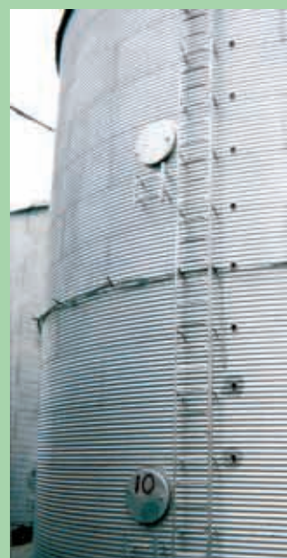
Barth put a window in every ring in each of his 10 bins. They're next to the ladders so they're easy to clean.
