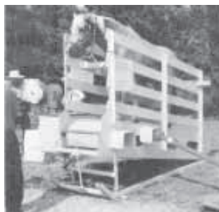
Horse-powered treadmill drives a pto shaft that can be used to perform a variety of jobs.
