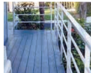
Tongue-and-groove 2 by 8 boards can be used as deck flooring.
