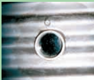
Bin windows are made from 3-in. pvc pipe, with one side covered by a piece of 1/8-in. clear plexiglas.
