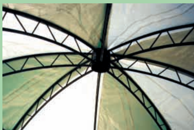
Secret to design of new domed building is the new center hub which joins conventional hoop-type trusses together.
