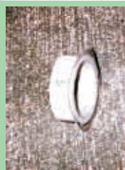
Bin windows are made from 3-in. pvc pipe, with one side covered by a piece of 1/8-in. clear plexiglas.
