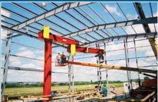
Installed in as little as two days
