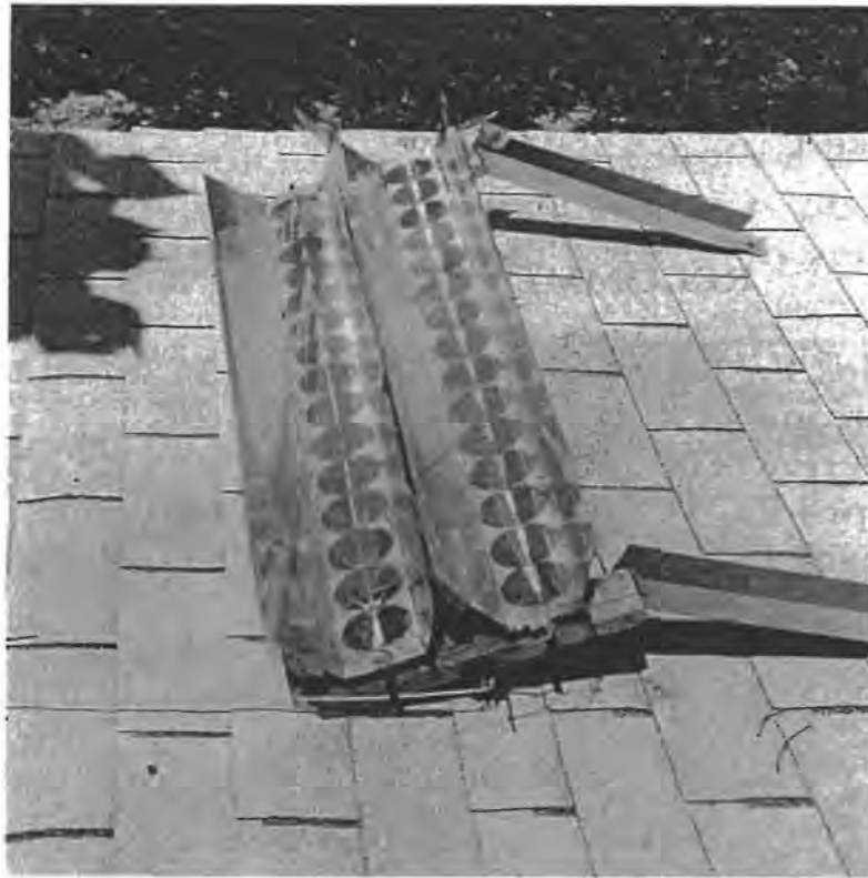
Figure 3.7. Trough-type parabolic collector, similar to that developed by Winston, mounted on the roof of the Raymond Frady residence near Miff- lin, Indiana. This type of hybrid concentrator photovoltaic system is particularly suitable for remote residential applications.
