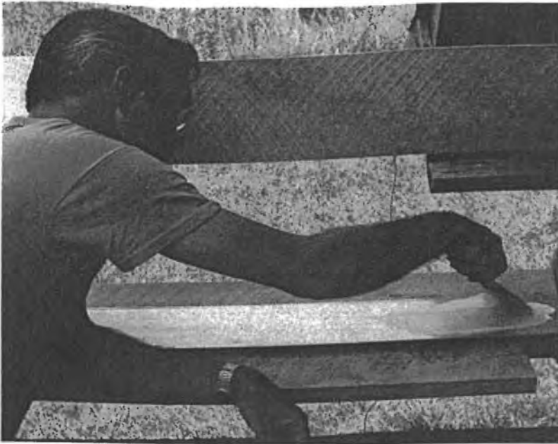
Figure A.8. Spreading silicone RTV caulk onto the backing plate.
