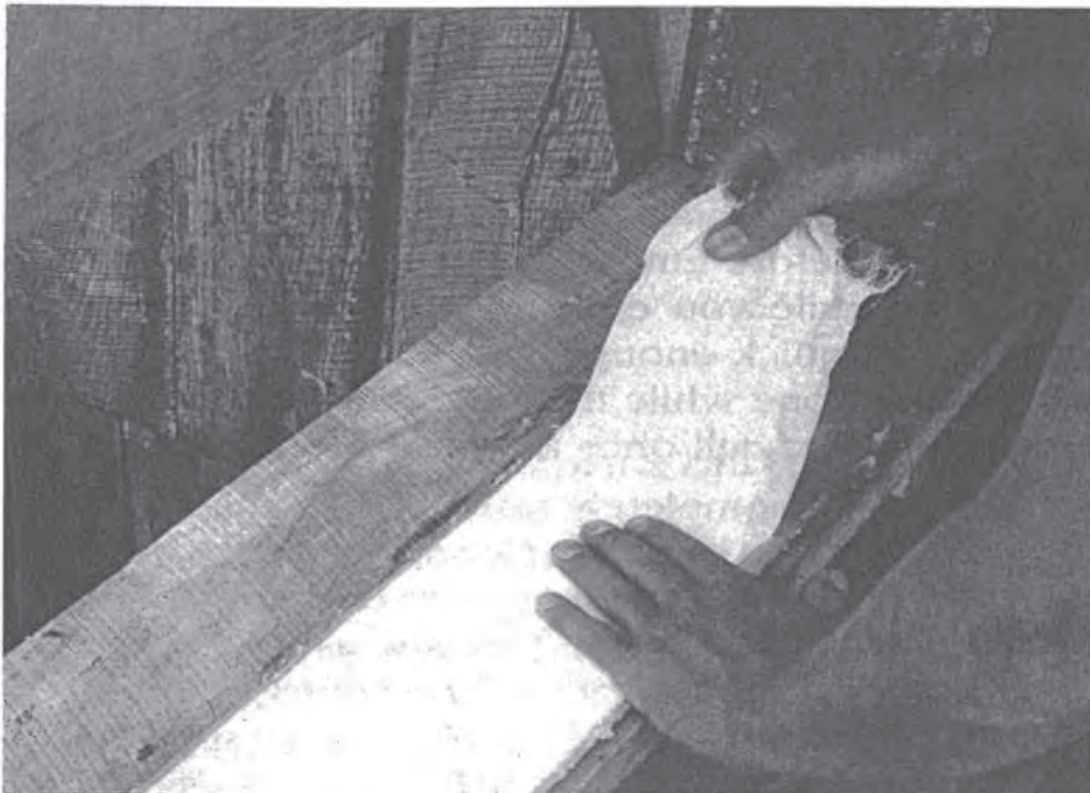
Figure A.9. Placing the cloth onto the fresh silicone. (Skyheat Workshop photo)
