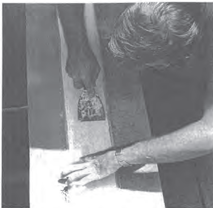
Figure A.10. Smoothing out a new layer of silicone over the cloth, completely embedding the cloth. (Skyheat Workshop photo)
