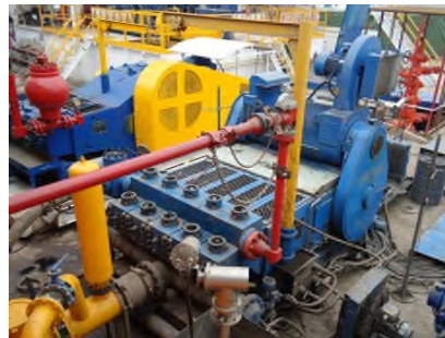
Test on drilling site
