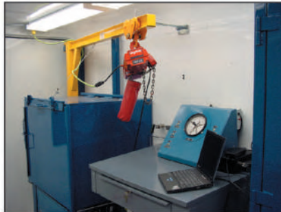
Pressure Test Station with full test capability to 30,000 psi; Inside test chamber for valves and integral connections.
