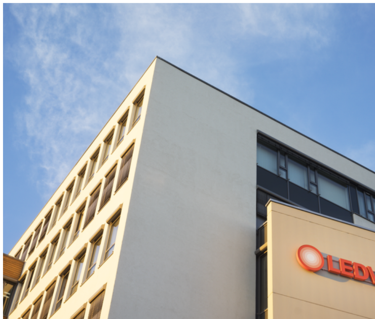
LEDVANCE Headquarters in Garching near Munich
