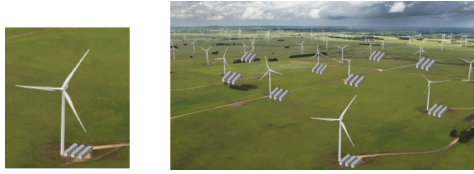
Figure 3. ZCCloud containers below wind turbines. Turbines can be several MW, and wind farms >250 MW.
