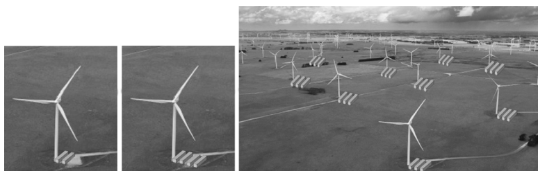
Figure 4: Scaling from Small: 1-container, 0.2 Petaflops, 0.05 MW, Medium: 4-container, 0.8 Petaflops both can be power by a single turbine. Large: 32-container, 6.4 PF, 1.6 MW, 1% of turbines in a wind farm
