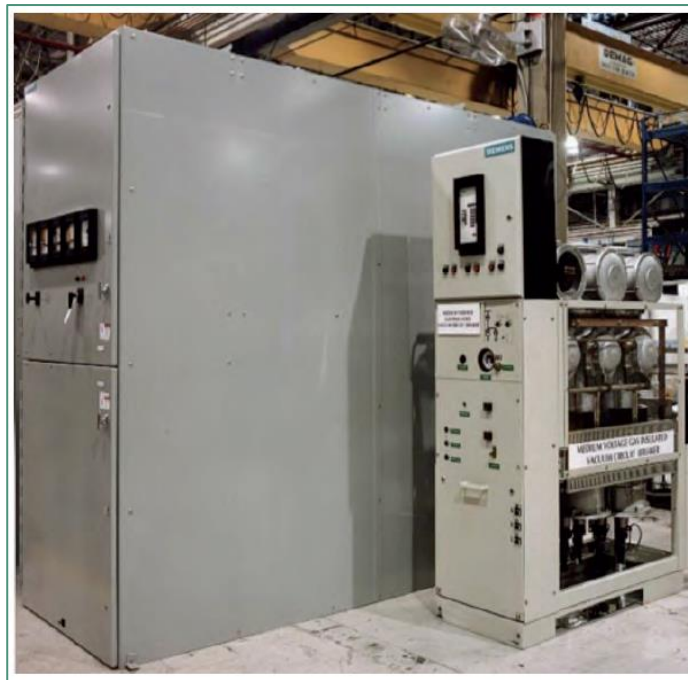
Figure 2-1: 36kV Indoor MV Switchgear comparison (AIS on left, SF 6 on right) [1]
