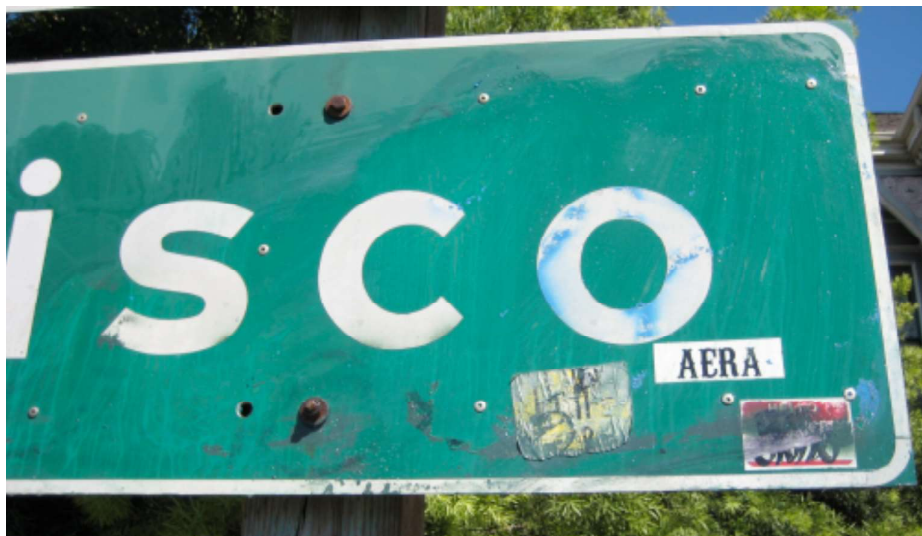
Figure 1-7: Older sign with non-reflective decals
