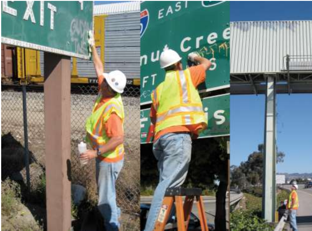
Figure 1-9: Methods of cleaning signs; far right requires a personnel lift
