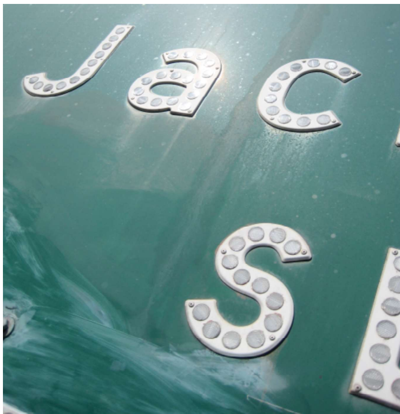
Figure 1-8: Older sign with reflectors in raised lettering
