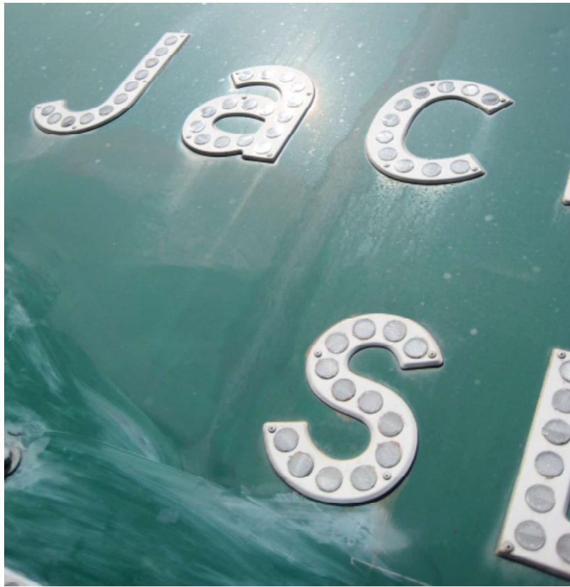
Figure 1-8: Older sign with reflectors in raised lettering
