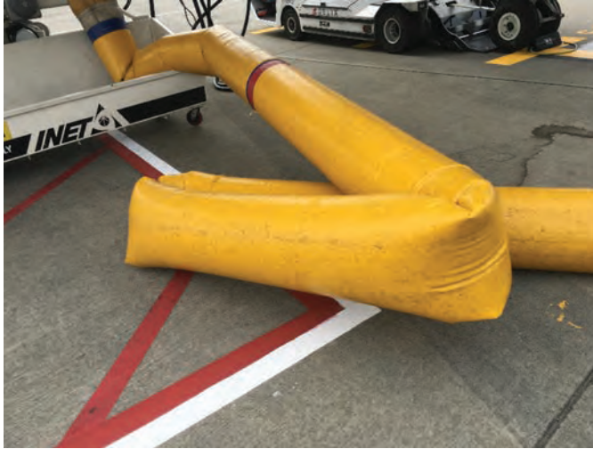
Figure 12. Kinked PCA hose (Source: Seattle–Tacoma International Airport).
