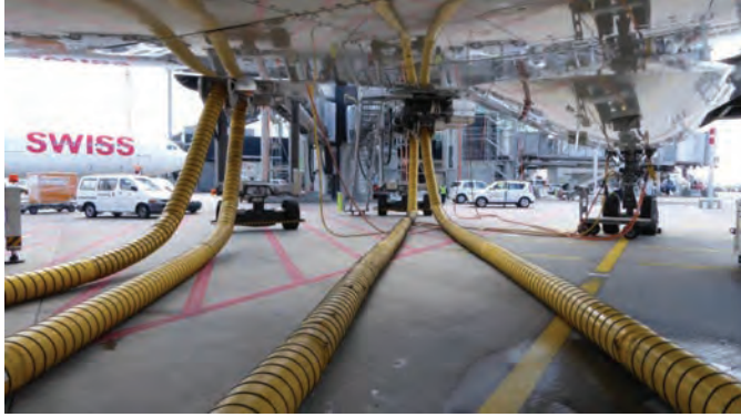
Figure 38. PCA hoses at Zurich International Airport (Source: Zurich International Airport).
