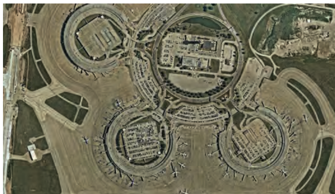
Figure 25. Aerial view of Kansas City International Airport terminals.
