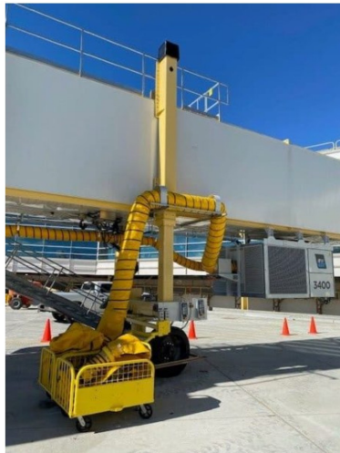
Trolley is connected with bogie and moves with the jet bridge
