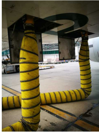
Wide body aircraft have two PCA receptacle. Two PCA hoses are connected with these aircrafts.
