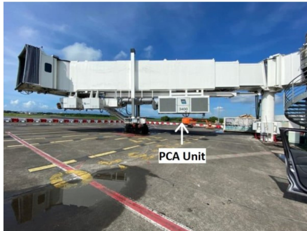
Bridge mounted PCA units generally hang under the bridge (Image Source: ITW GSE )
