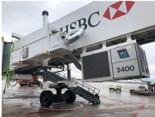
Bridge mounted PCA units save space on the ramp (Image Source: ITW GSE )
