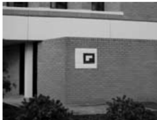
Figure 3: Fiducial marker on a building
