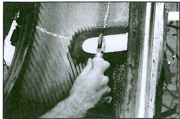
27 Stitch the platform into place using a Tech stitcher.
