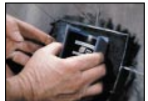
Install the repair unit.
