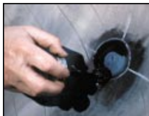
Apply 76 Repair Sealant over the entire buffed area and repair.
