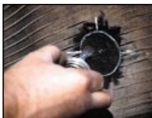
Apply the Special Blue Cement; continue brushing until it is dry.
