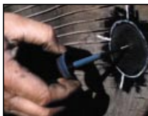
Install the Minicombi or RemaStem
