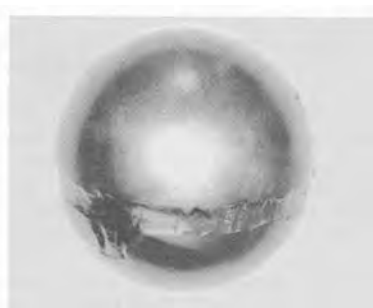
FIGURE 15 Erosion damage of an AISI-type, 440C stainless steel ball valve in a coal slurry service
