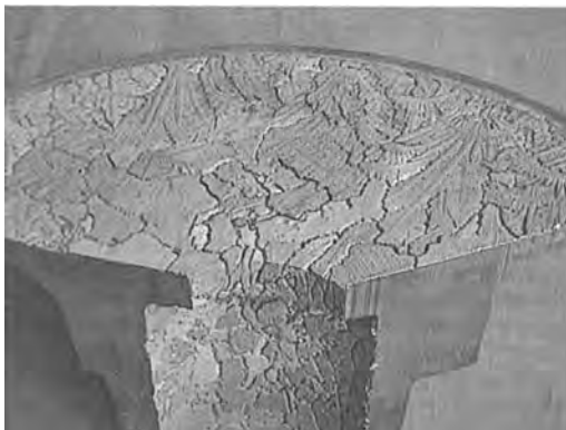
FIGURE 7 The surface of a stuffing box cover that experienced intergranular corrosion due to sensitization. The grains are clearly evident on the interior of the bore as well.
