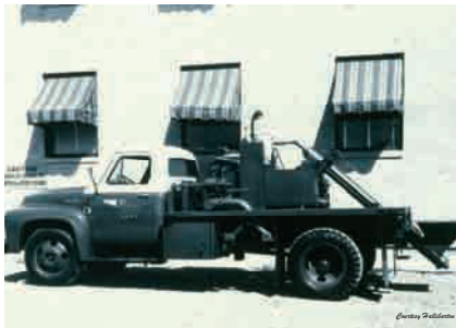
Fig. 4 —Early screw-type sand blender.
