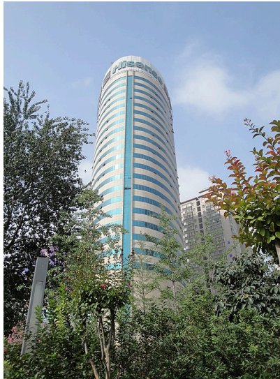
Headquarters in Qingdao, Shandong
