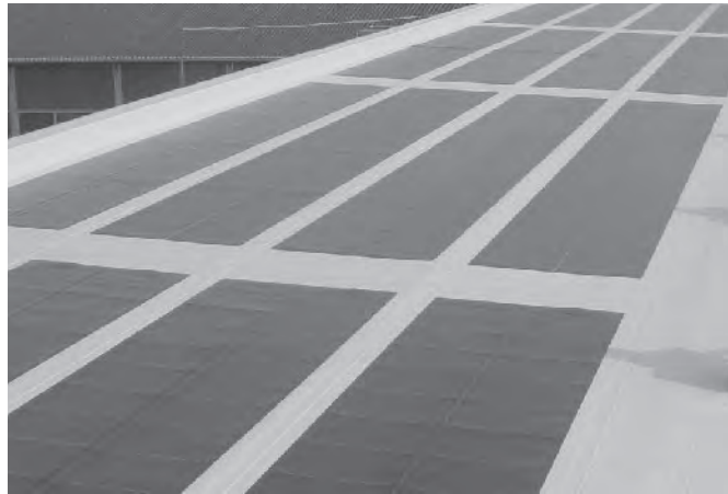
Figure 22.36 Alwitra Evalon® roofing foil with amorphous silicon cells. Reproduced with permission by O.O. Energiesparverband
