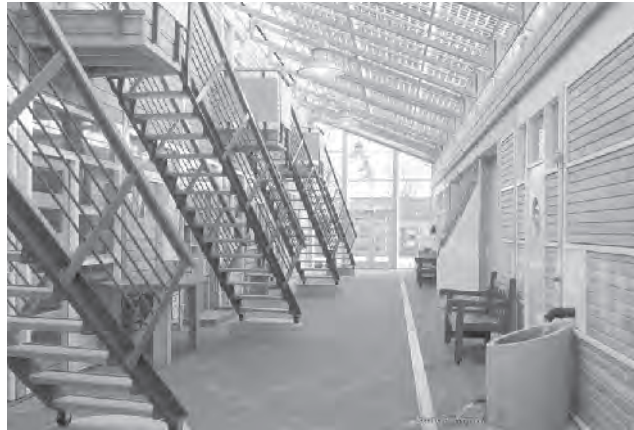
Figure 22.14 Corridor in the Centre for Sustainability De Kleine Aarde in Boxtel (NL). The space is unheated and naturally ventilated. The 6.7 kWp PV system with transparent modules has a double function and reduces the heat load by around 70%. Reproduced from Reijenga T, Bottger W, Proc. 2 nd WC Photovoltaic Solar Energy Conversion , 2748–2751 (1998) with permission by NOVEM, R Schropp [11]
