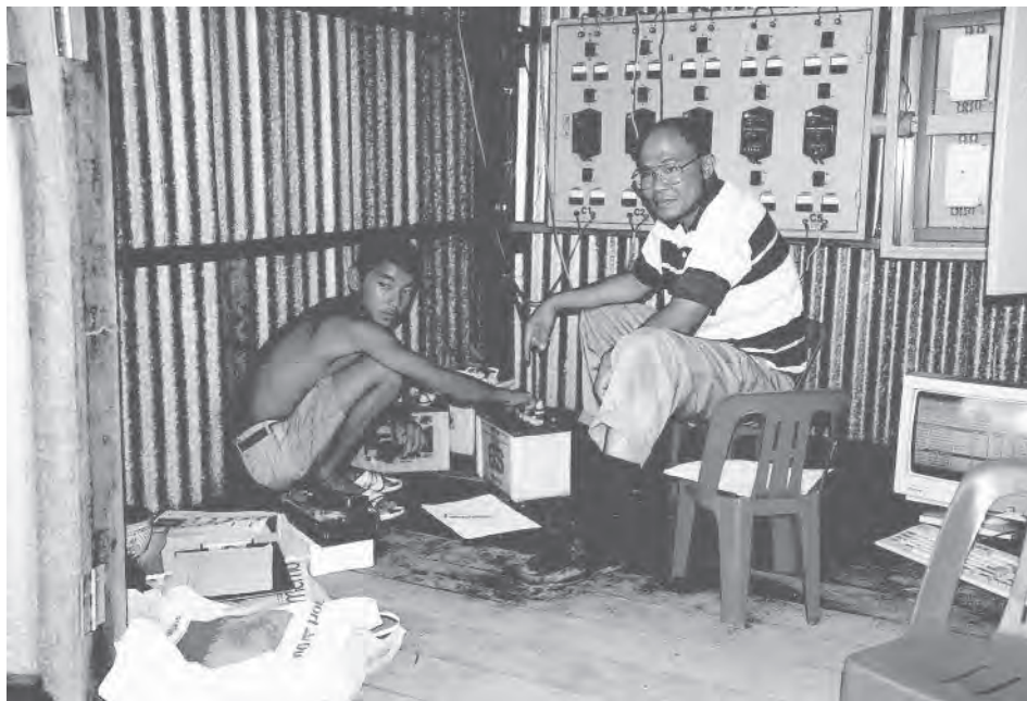
Figure 17.11 A typical PV powered battery-charging station in rural Thailand (Source: Fraunhofer ISE, Freiburg [14])
