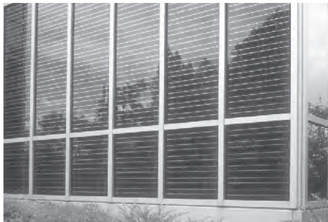
Figure 22.37 Schuco 1.9 kWp roof profile system with transparent modules in the Energy Forum Center in Bad Oeyenhausen (D). This mounting system can also be used in (difficult) horizontal situations. Reproduced with permission by BEAR Architecten T. Reijenga
