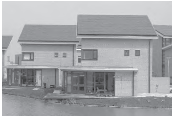
Figure 22.34 Alutec profile system in a new roof in Langedijk HAL (NL). Capacity of the system is 53 kWp and the project is part of the 5 MW BIPV project. Reproduced with permission by BEAR Architecten M. van Kerckhoven
