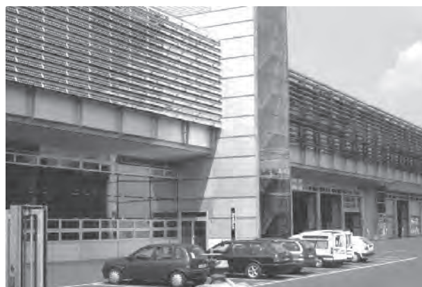
Figure 22.9 Colt shading system that is optimized for sun control. The distance between the louvers with PV modules cause shading on 50% of the PV cells; 47 kWp PV system at Stadtwerke in Winterthur (CH). Reproduced with permission by BEAR Architecten T. Reijenga
