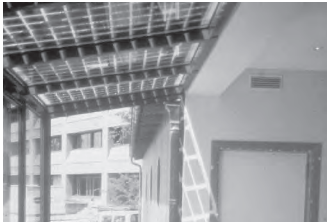
Figure 22.26 The canteen at the IMEC in Leuven (B) has an entrance with attractive-looking transparent modules in the roof. Reproduced with permission by IMEC
