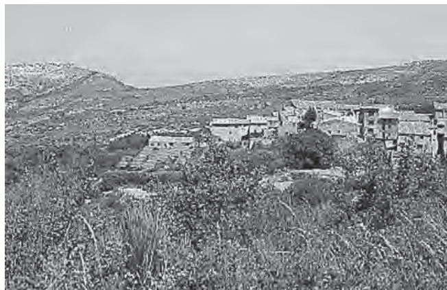
Figure 17.15 PV-Diesel-Hybrid system in Llavería (Source: TTA, Barcelona)
