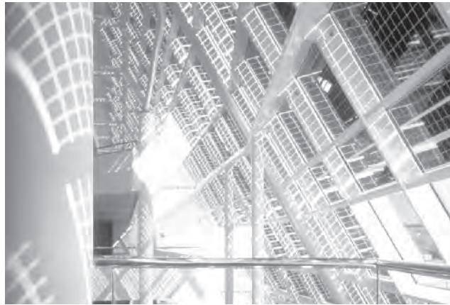
Figure 22.4 Solar office in Doxford Sunderland (UK) with a transparent double-glazing PV system integrated in the facade. The 73 kWp PV system is manufactured by Saint Gobain and mounted in Schuco window frames. Reproduced with permission by Dennis Gilbert
