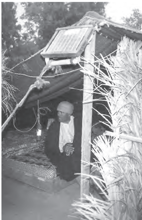
Figure 17.5 Photovoltaically powered light in a hut in Tunisia (Source: Ludwig-Bolkow-Stiftung, Ottobrunn)
