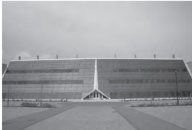
Figure 22.18 The Schuco facade in the Solar office in Doxford, Sunderland (UK) is well engineered. Reproduced with permission by BEAR Architecten T. Reijenga
