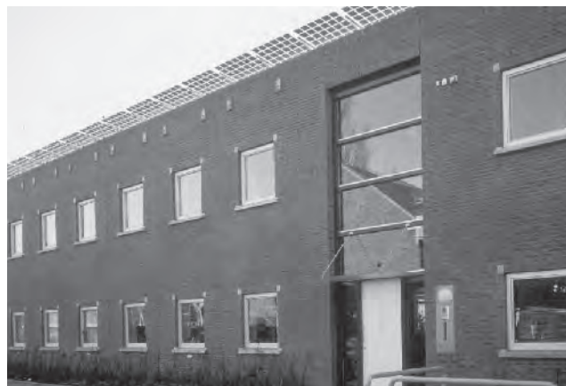
Figure 22.24 In this office building in Gouda (NL), the 6.2 kWp PV system is mounted on top of the facade as a canopy that protects the wall. The architect's intention was to show the PV system to his clients when they visit the office. Reproduced with permission by BEAR Architecten T. Reijenga
