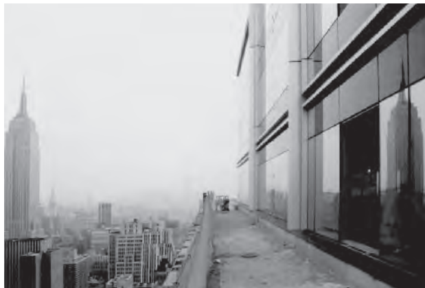
Figure 22.2 Integrated facade system with 14 kWp amorphous silicon modules made by Energy Photovoltaics (EPV) in New Jersey, USA on top of a skyscraper at Four Times Square, New York, USA. The PV modules are the dark regions on the facade near the top. Reproduced from Kiss G, Proc. 2 nd WC Photovoltaic Solar Energy Conversion , 2452–2455 (1998) with permission by Gregory Kiss [7]
