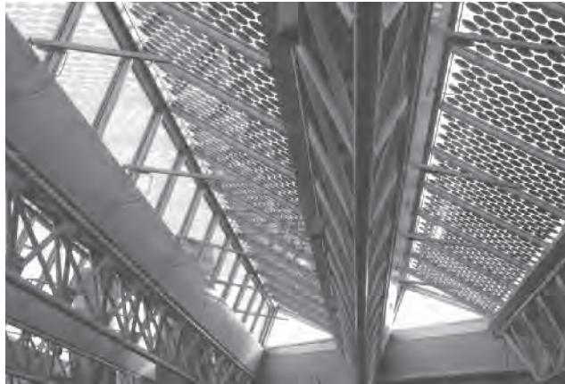
Figure 22.31 Atrium roof of the Brundtland Centre building from the inside. Because the saw-tooth roof casts a shadow on the modules, some of the cells are fake. This solution achieves a more elegant look from the inside. Reproduced with permission by BEAR Architecten T. Reijenga
