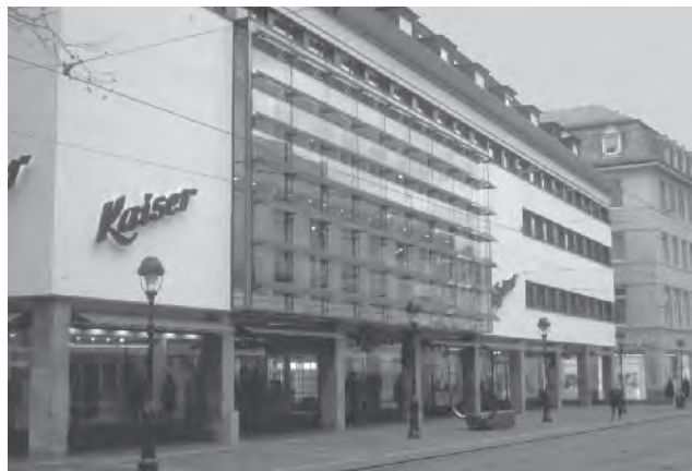
Figure 22.10 Daylight control at the Kaiser fashion house in Freiburg (D). This 4 kWp PV system on louvers is mounted in front of the glass facade and prevents glare inside. The PV louvers are in the center of the figure. Reproduced with permission by BEAR Architecten T. Reijenga
