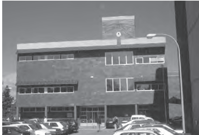
Figure 22.21 The IES building in Madrid (E) has a 6.6 kWp PV system that was added shortly after the building was finished. The modules are mounted on the facade above the windows and keep out the sun. Reproduced with permission by BEAR Architecten T. Reijenga
