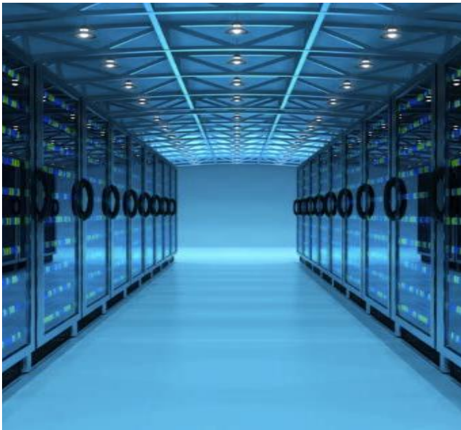
Optical Data Center Interconnect
