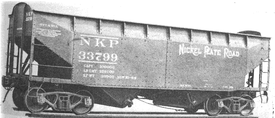
Fig. 2.621—New York, Chicago & St. Louis (Nickel Plate) 50-ton twin hopper coal car. Builder, American Car and Foundry Co. Light weight, 33,900 lb.; load limit, 129,100 lb.; capacity, 2,081 cu. ft.; inside, length 33 ft. 0 in.; width 10 ft. 4 in.; height of sides 10 ft. 6 in.
