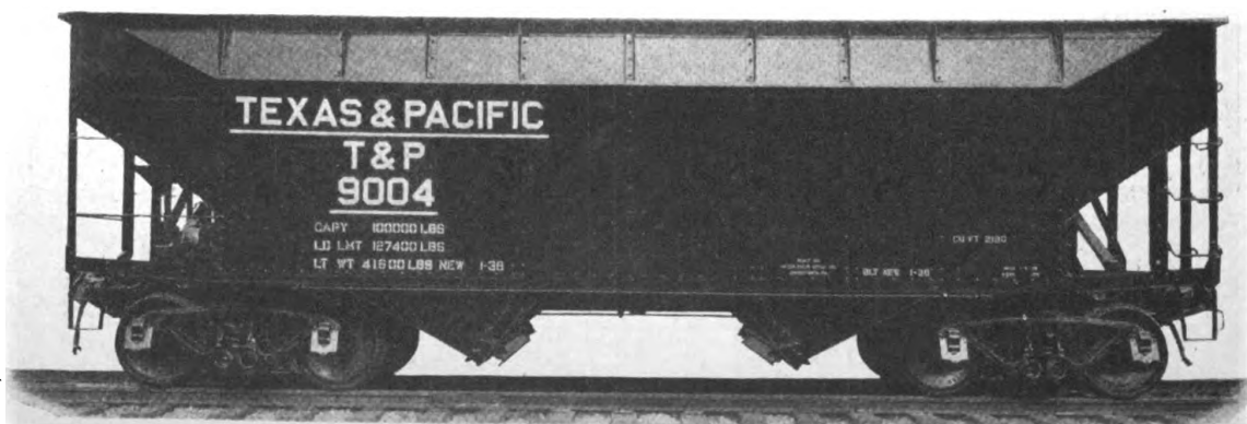
Hopper car built new with Wine Cast Steel Hopper Frames
