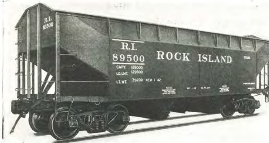
Fig. 2.613—Chicago, Rock Island & Pacific 128,000-lb. capacity twin hopper coal car. Builder, American Car and Foundry Co.
