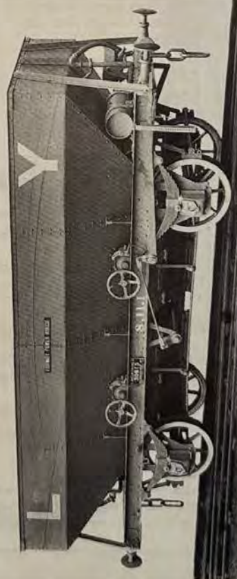
Plate 205. The official photograph of wagon No. 30813 as built and painted in June 1904. The undergear had been left grey for photographic purposes. The triangular fillets supporting the angled sides show up well.
