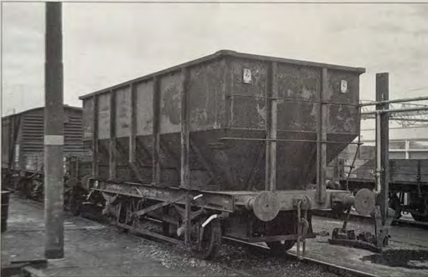
B337235 at Hoo Junction, Rochester in December 1968. This lot 3466 wagon is in such a rusty condition it is difficult to work out the livery. It should be grey and does not appear to have ever been repainted. Tare weight: 10ton 14cwt. (Author's Ref No W1081/DL)
