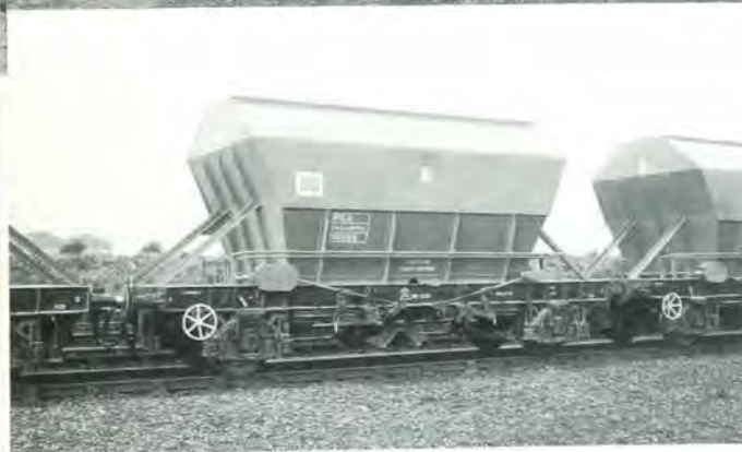
The automatic door-operating mechanism can be clearly seen in this view of BSTE 18058, taken at Tees Yard in September 1987. Note the lack of prefix letters on the vehicle's data panel, a feature common to this fleet. Originally painted a pale green, these wagons were being repainted in the grey and black livery illustrated here, with blue and white British Steel symbol.
