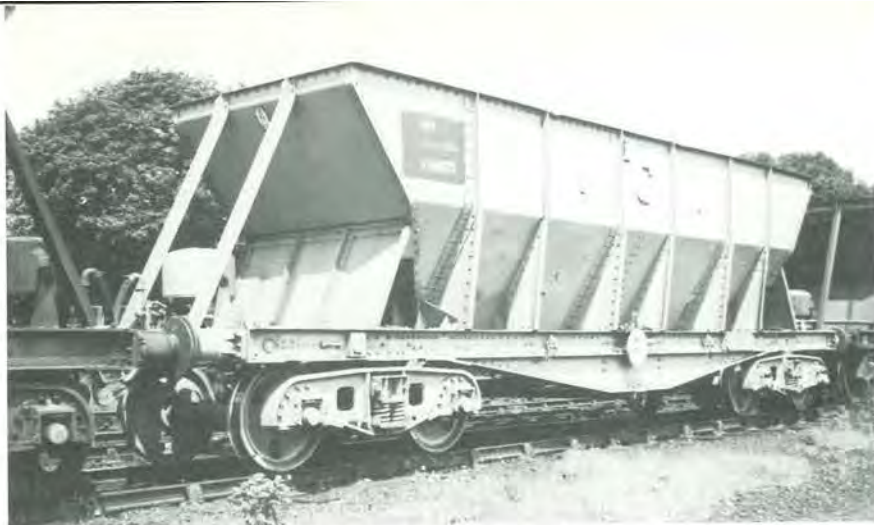
Above ICIM 19129, one of the Charles Roberts-built limestone bogie hoppers, photographed at Northwich in August 1987. Apart from the addition of roller bearings, this wagon remains in virtually its original condition, although it has recently been repainted pale grey with the number panel in white on a black ground. Note the raised 'ICI' letters on the side; an earlier version of the livery had these painted orange.
