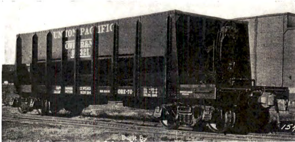
Fig. 2.672—Union Pacific (O.-W. R. & N.) 70-ton ore car, AAR Class HMA. Builder, St. Louis Car Company. Light weight, 62,300 lb.; load limit, 147,700 lb.; capacity, 1,360 cu. ft.; inside, length 28 ft. 0 in.; inside, width 9 ft. 6 in.
