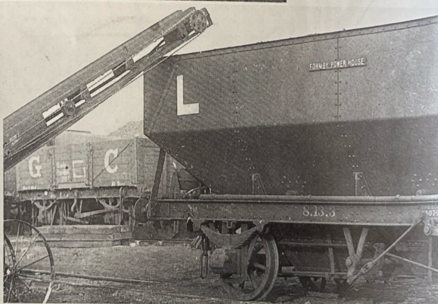
Plate 207. A posed shot at Clifton Junction Power Station in September 1919 with S35 Order wagon No. 30790 still lower height but redesigned for 'Clifton Power Station'. The wagon tared at only 7.19.1 and had a lovely repair on the nearest corner. Fully laden, its buffers seem dangerously lower than those of battery electric loco No. 2. NATIONAL RAILWAY MUSEUM
