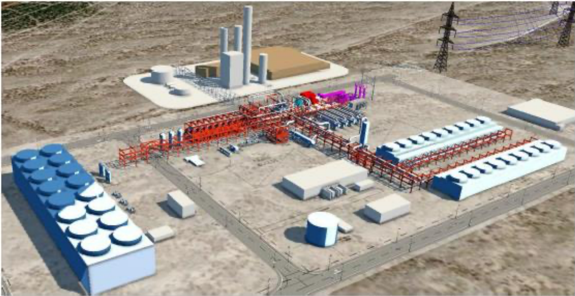
Figure 2: NET Power nominal 300MWe Commercial Plant Concept
