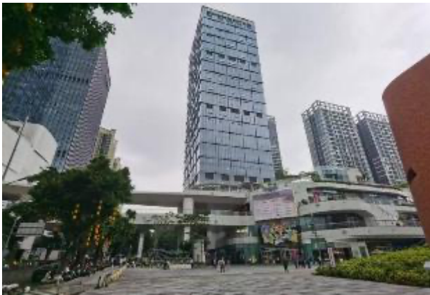
Figure 9 Outside View of the Building
