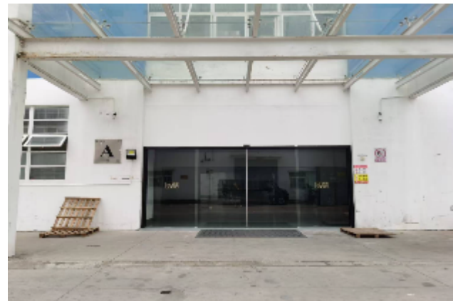
Figure 16 Entrance of Building A
