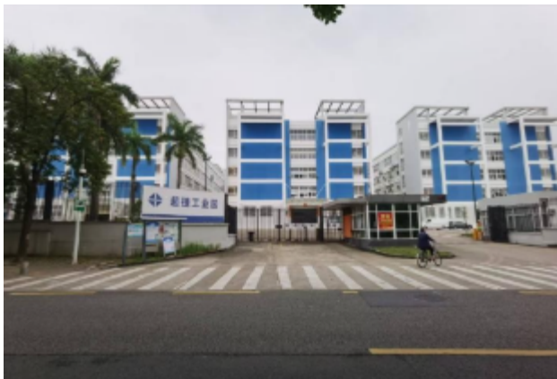
Figure 15 Outside View of the Industrial Park
