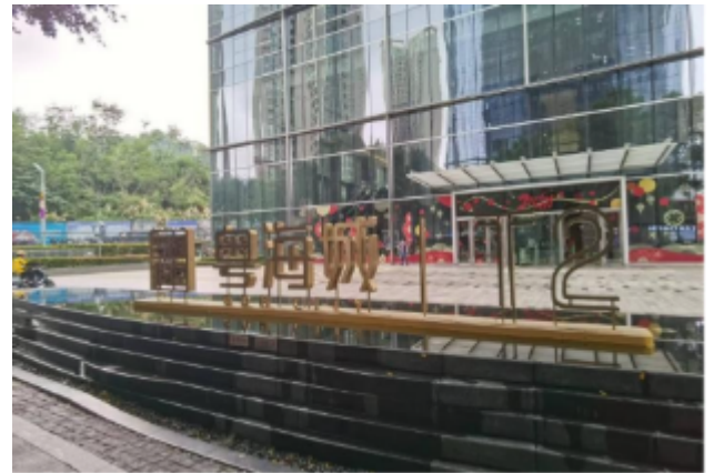
Figure 10 Outside View of the Building
