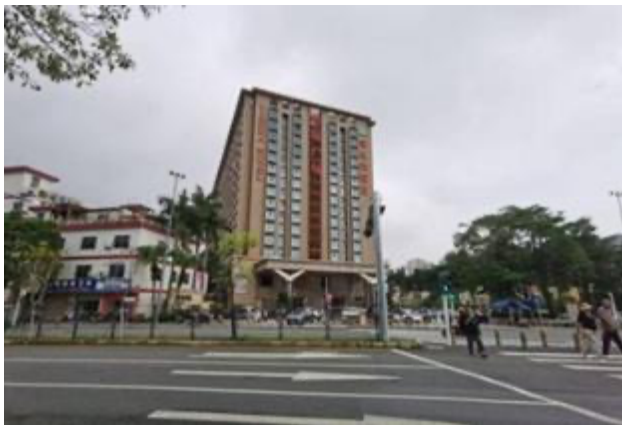
Figure 1 Outside View of the Building
