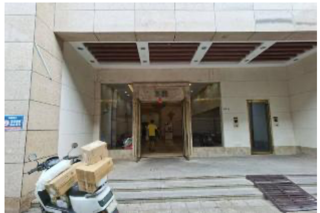
Figure 2 The Entrance of Building B
