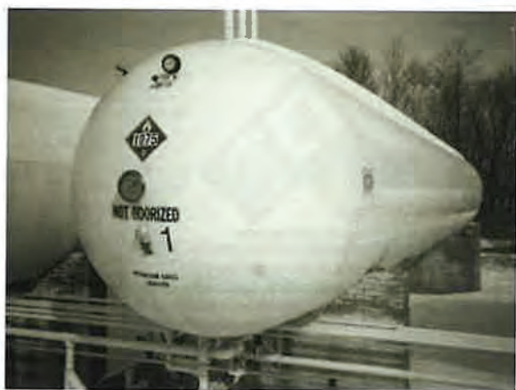
EXHIBIT 5.18 ASME Containers Marked NOT ODORIZED.
