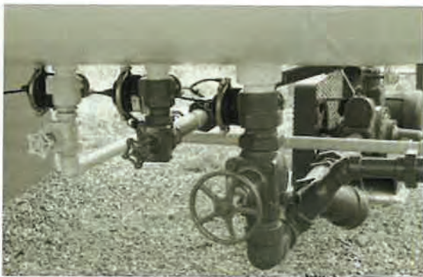
EXHIBIT 5.44 ASME Container with Labeled and Color-Coded Connections. (Courtesy of Propane Education and Research Council)
