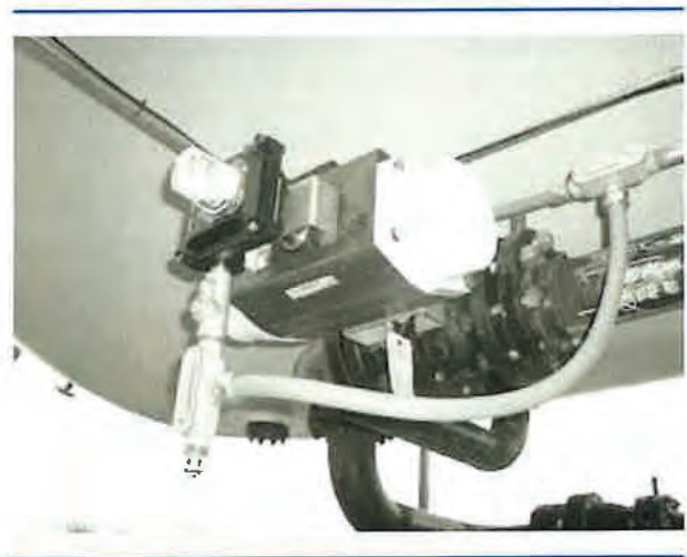
EXHIBIT 5.34 Tank Valve Complying with API 607. (Courtesy of Superior Energy Systems)
