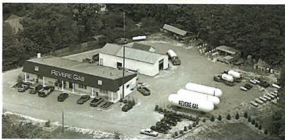
EXHIBIT 3.2 Aerial View of a Bulk Plant. (Courtesy of Revere Gas and Appliance)
