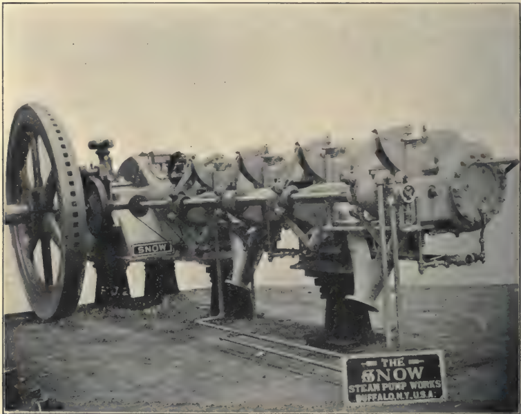
FIG. 12-72. — Snow Type B Gas Engine.
