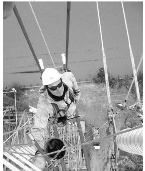
Samson's LightSpeed-3 is a dielectric 3-strand rope utilizing high-tenacity monofilament polypropylene fibers with an advanced coating solution.
