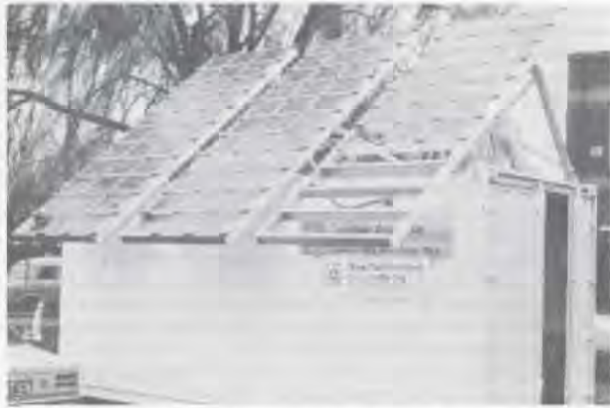
Figure 13.10. Solar power supply designed to provide approximately 100 to 150 W of electrical power continuously for a microwave repeater station. The shipping container supports the solar modules, as well as housing the storage batteries, control electronics, and facilities for servicing crews. (Photograph courtesy of Telecom Australia.)
