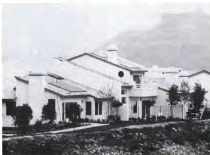
These Laguna Del Mar townhomes use PV to supply part of their electricity. They also use the local utility as a backup to store any extra power they may produce. An extra meter on each home monitors the electricity fed back to the utility company.
