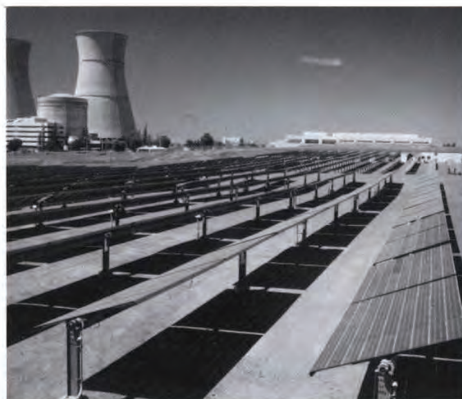
As the cost of photovoltaics continues to decrease, the technology becomes increasingly competitive for utilities. Above is a 2-MW single-axis-tracking photovoltaic system at Sacramento Municipal Utility District's Rancho Seco facility in Sacramento, California.
