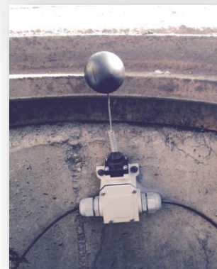
Figure 7. Vertical wall installation
