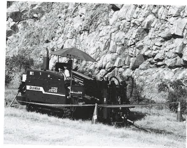
FIGURE 12.9 A horizontal directional drilling (HDD) machine in operation. (Courtesy of Ditch Witch Company.)
