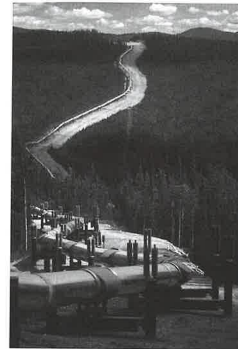
FIGURE 1.3 An aboveground portion of the Trans-Alaska Pipeline about 5 mi north of the Yukon River. The pipeline was designed to meet the most stringent environmental standards for protecting the arctic environment. (Courtesy of Alyeska Pipeline Service Company.)
