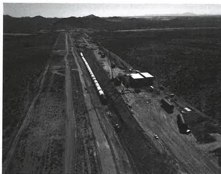
FIGURE 1.4 One of the world's largest diameter concrete pipes (21 ft I.D.) used by the U.S. Bureau of Reclamation to convey water as a part of an aqueduct in central Arizona. (Courtesy of Bureau of Reclamation.)
