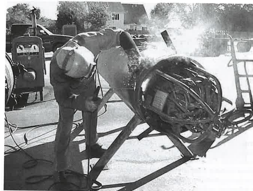
FIGURE 12.6 At the National Pipeline Welding School in Tulsa, Oklahoma, operated by American Pipeliners Union Local 798, instructor Gary Allison demonstrates how to weld a 24-in steel pipe using an electric arc and an internal lineup clamp. (Courtesy of Local 798.)
