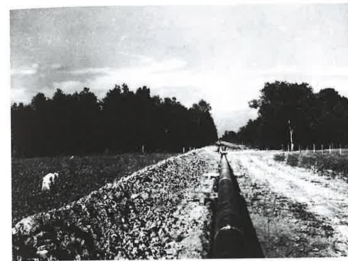
FIGURE 1.1 The Big Inch pipeline under construction in 1942; historic photograph showing the pipeline crossing a cotton field near the Arkansas–Missouri border. (Courtesy of Duke Energy.)
