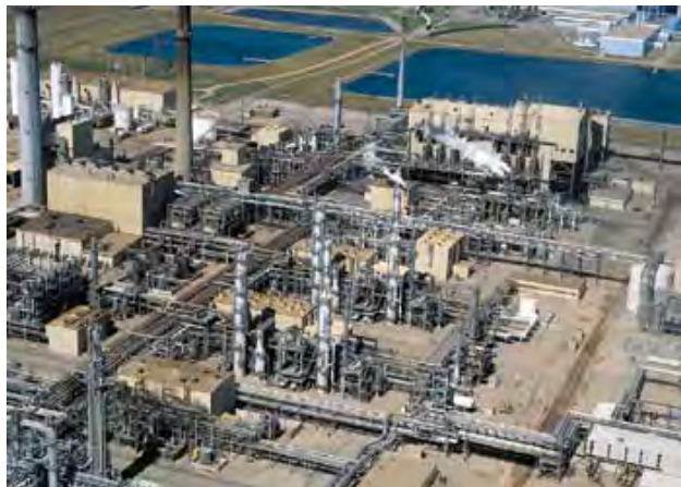
Figure 3.15 North Dakota coal gasification plant with 3.3 MtCO 2 yr -1 capture using a cold methanol, physical solvent process (cluster of 4 tall columns in the middle of the picture represent the H 2 S and CO 2 capture processes; part of the captured stream is used for EOR with CO 2 storage in Weyburn, Saskatchewan, Canada).
