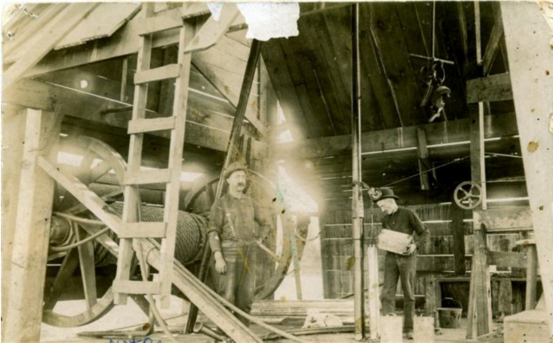
Pouring nitro into a canister to prepare a “shooting” of a well drilled using a cable-tool rig powered with a nearby steam boiler.
