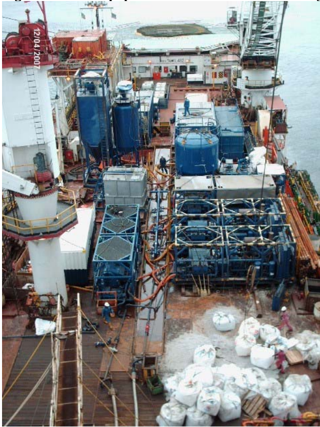
Figure 2 – Frac Equipment on Barracuda Tender Barge
