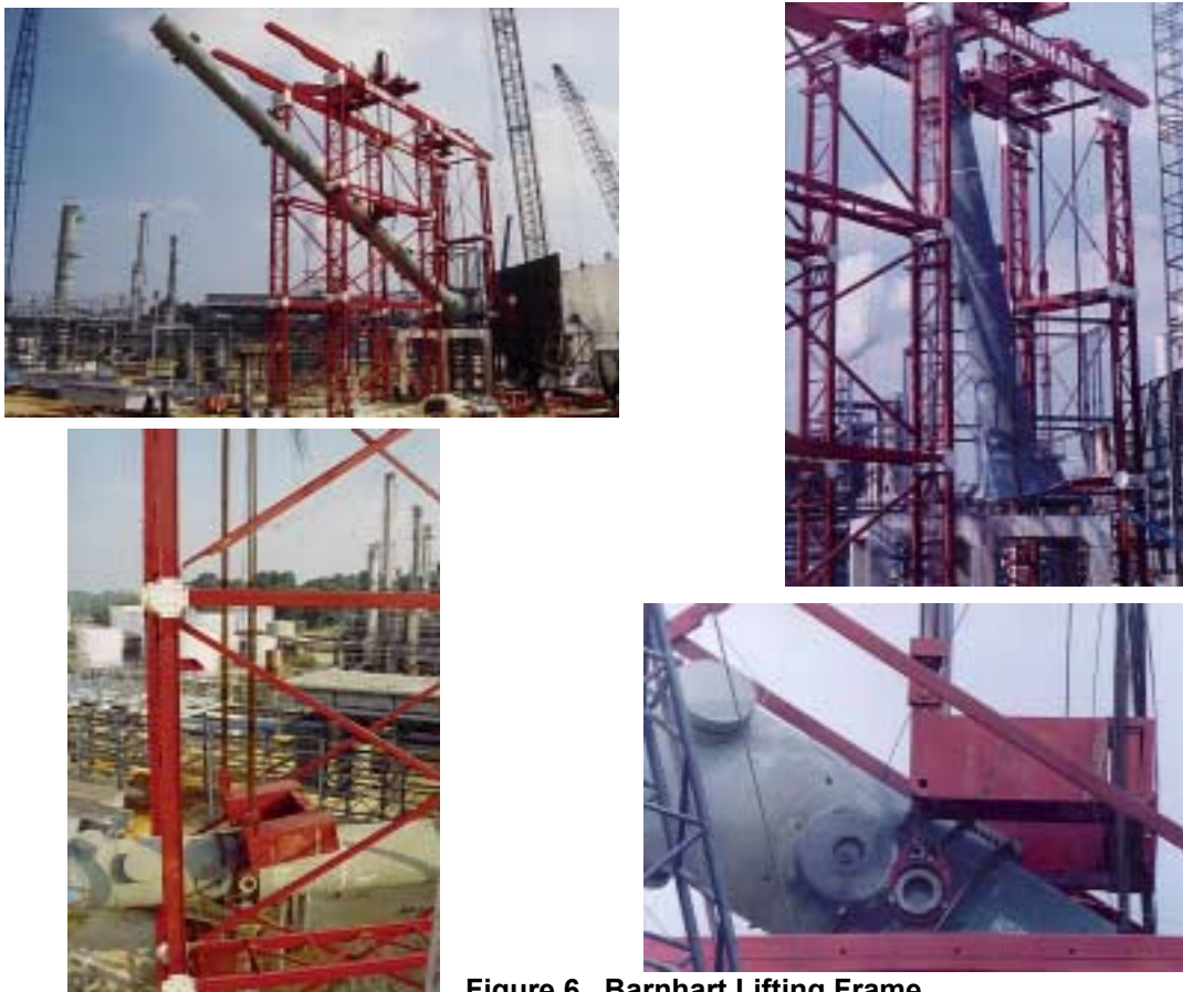
Figure 6. Barnhart Lifting Frame
