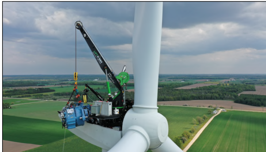
LiftWerx RotorHook https://liftwerx.com/our-cranes/
