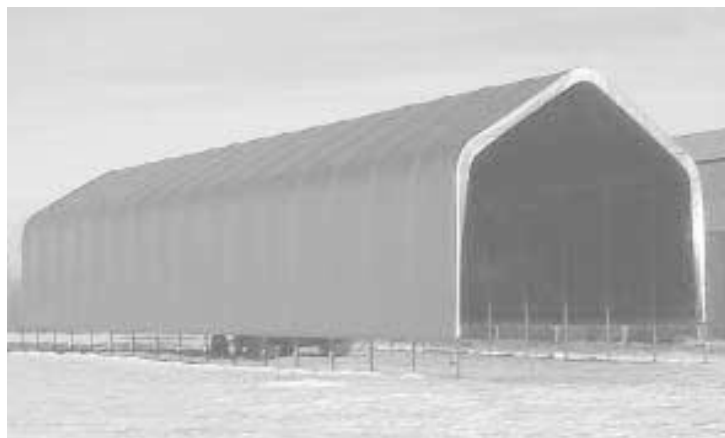
Shelter is 27 ft. wide by 96 ft. long by 25 ft. high and holds 26 typical bale wagon stacks. Roof's pitch allows snow to slide off before any accumulation can put stress on cover.
