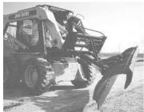
Shrum mounted a plate on skid steer loader in place of bucket, then fitted it with a snowplow designed for a pickup.
