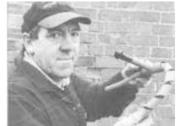
Alan Hughes and his spiral pipe cutter. "walks" the tool along the pipe. When you've cut enough pipe, you just withdraw the blade and slip the tool off. (Alan Hughes, Home Farm, Berwick, Shrewsbury, Shropshire, England)
