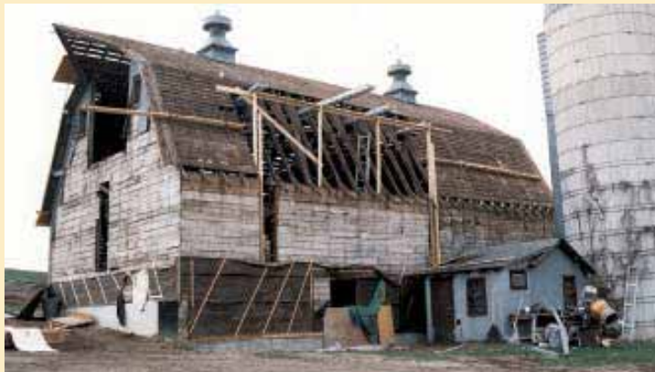
This photo was taken after the original cedar roof and galvanized tin siding had been removed.
