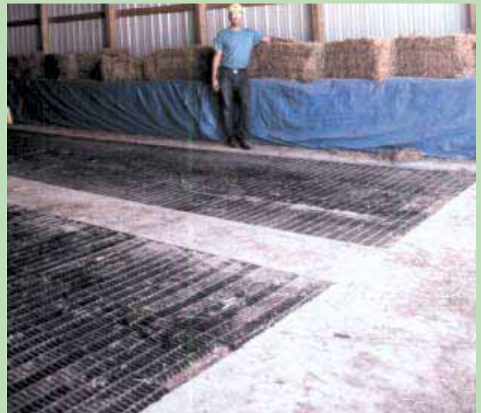
Building has a concrete floor with inset metal grates. Two 50-ft. long, 7-ft. wide tunnels beneath floor bring in warm air delivered by fan.
