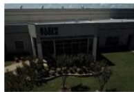
Mansfield, TX • USA
