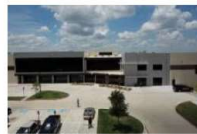
Mansfield, TX • USA
